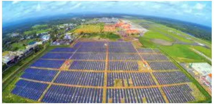
Solar Generator in Cochin Airport
