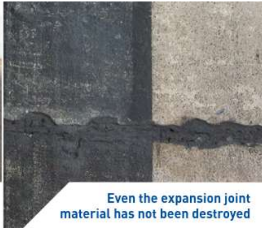
Cleaning results on concrete runway
